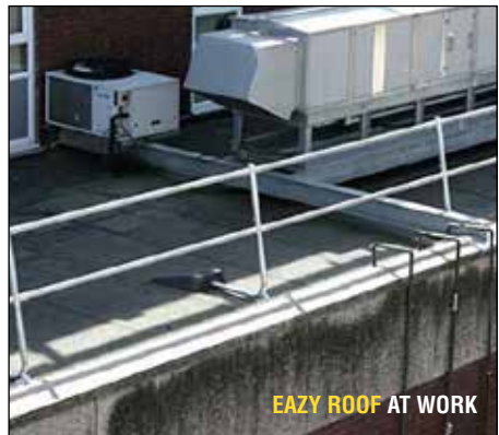
EAZY ROOF AT WORK
